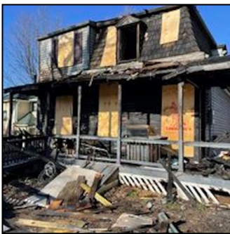
After the fire. HFI photo
